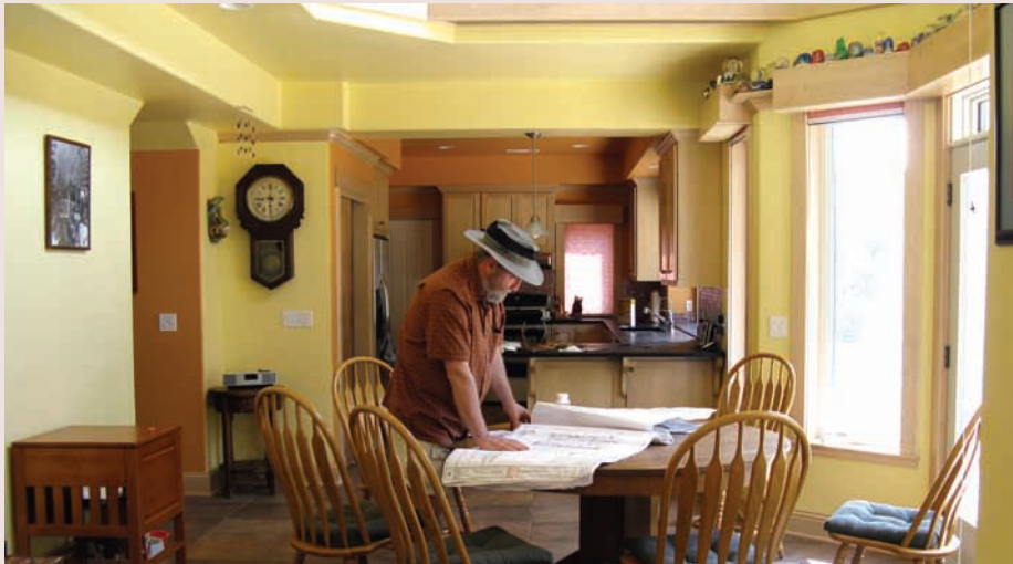
Andy Kerr looking over the house plans at the table; Indirect summer south light bathes the room. Solar thermal mass in floor and in wall to the rear of the eating area. Credit: Karen Chase
